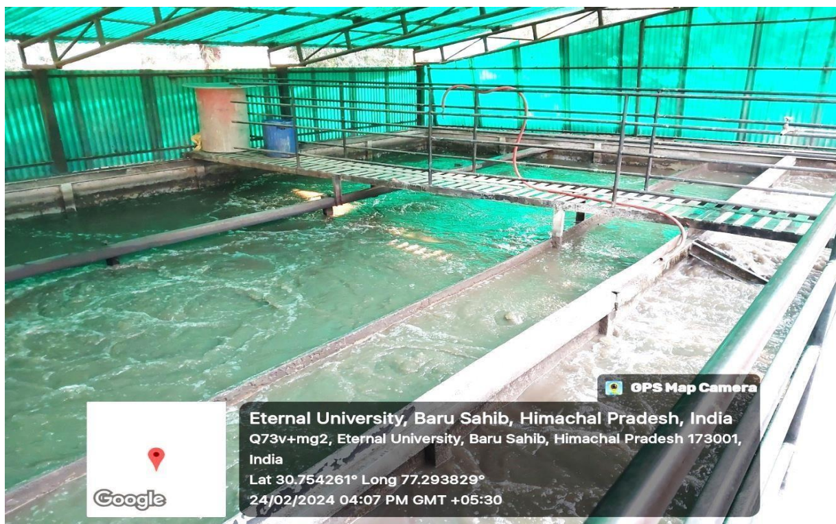
Sewage Storage Tank and Safe Reactor
