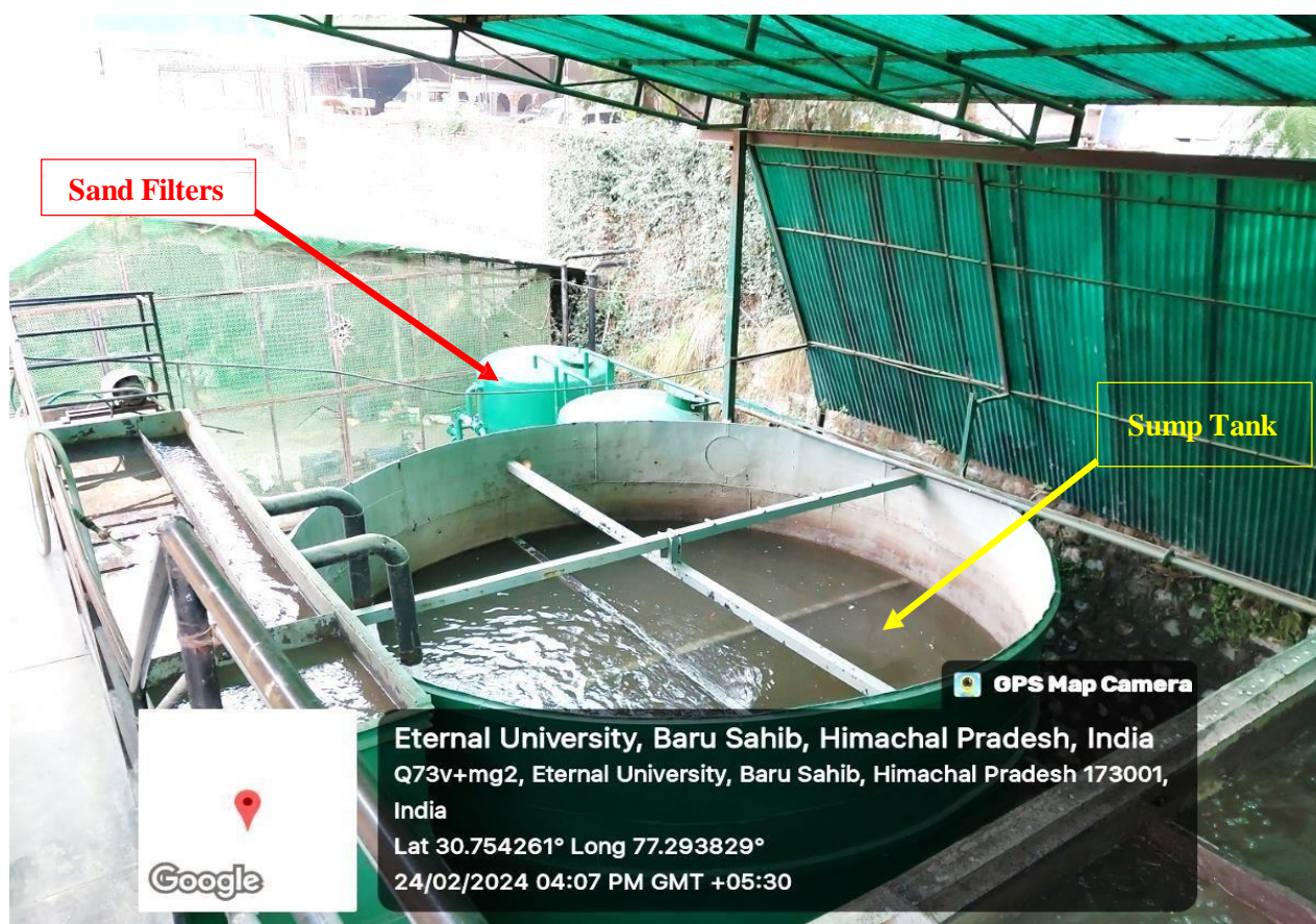
Sump Tank and Sand Filter
