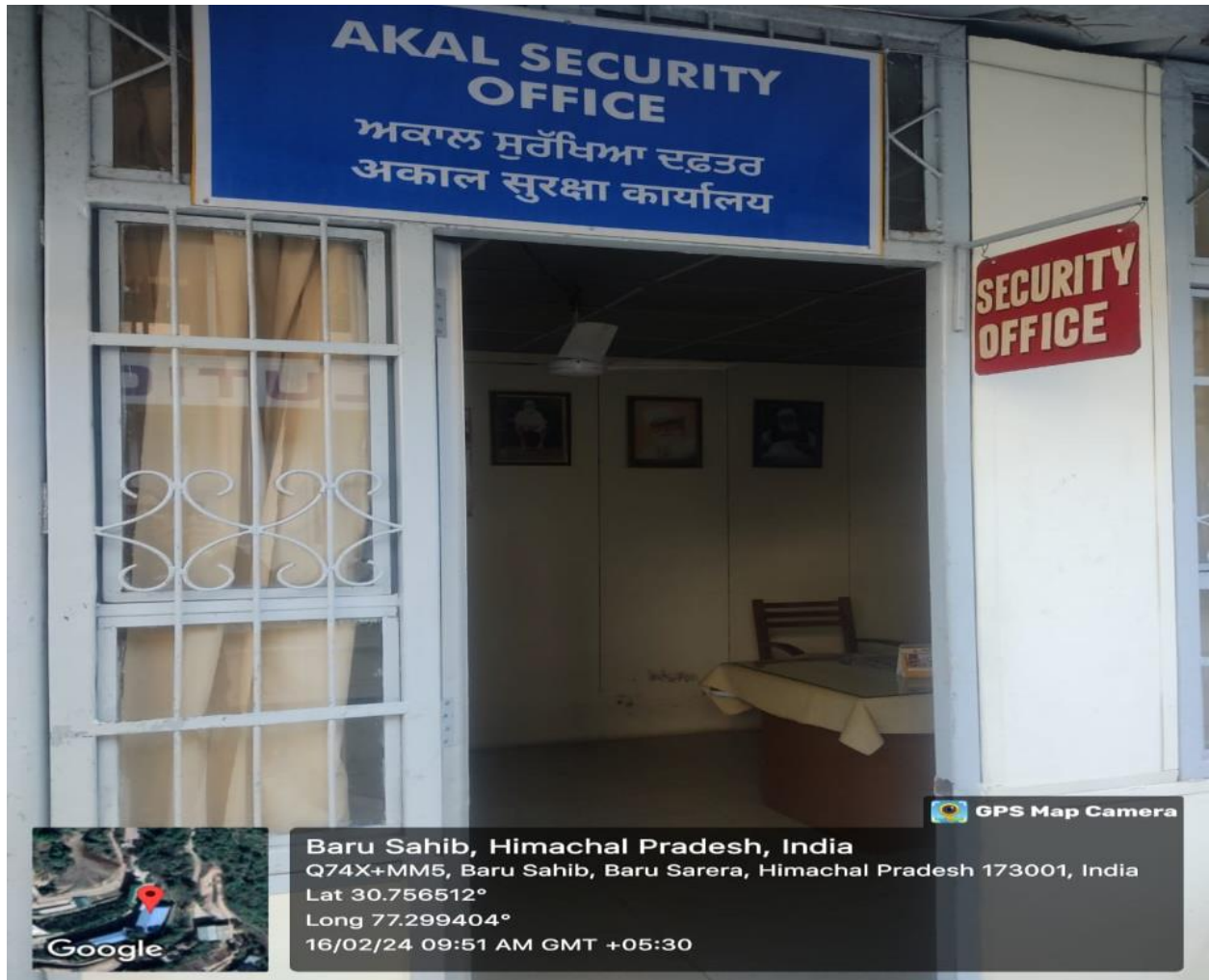
Security Office, University Barrier
