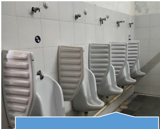
Waterless Urinals to Save Water
