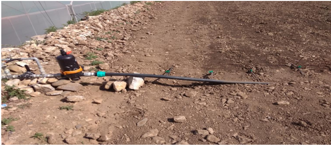
This photograph showing the installation of main line of subsurface drip irrigation with water filter, venturi injector and control valve
